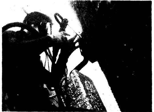
Fig. 6. Underwater Welding of galvanic anode.
